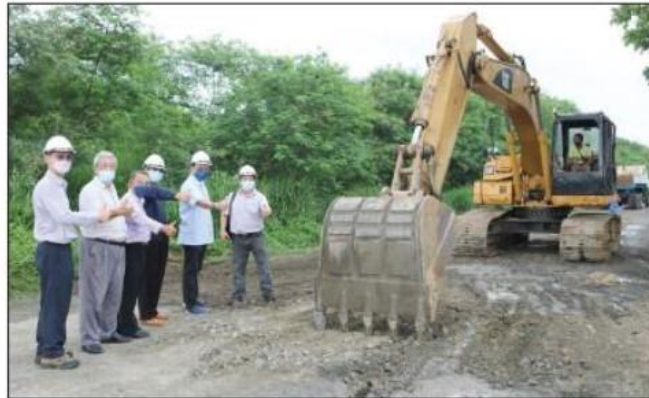
Gan (fifth from left) on the site to observe road repair and upgrading works in POIC Lahad Datu.
